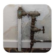
A 'spread-out' damp area at low level may indicate that the DPC has been 'bridged' by raising the level of external pavings or soil, which allows groundwater to bypass the DPC and enter the wall above it. The remedy is to lower the ground level again, so the edge of the DPC is visible, ideally at least 150mm (two brick courses) above ground.
