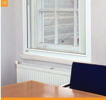
Secondary glazing reduces heat loss while retaining the existing window and its external appearance. (Photograph courtesy of English Heritage)
